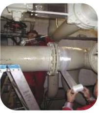
301 Epoxy Resin Hardener was brush applied to pipework situated in a plant room. The pipe wall thickness had deteriorated over time and the pipes were weeping hot water onto the floor below, Due to the fragile state of the pipes surface preparation was carried out using hand held wire brushes. Once the surface of the pipe had dried 301 Epoxy Resin and Hardener was applied at 1mm wet film thickness to the pipe surface and wrapped 3 times using 100mm glass tape
