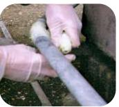
A chemical process line had started to leak due to a hole forming in the pipe wall, the surface was mechanically abraded and 108 Pipe Repair Tape wrapped around the pipe work to a minimum thickness of 12mm over the repair area.
