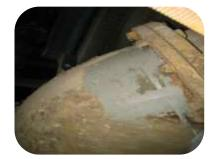
A hot chemical process line operating at 50° C was leaking around the flange fitting. He onsite contractor mechanically abraded the leaking pipe surface and cold bonded a steel plate to the repair surface. The steel plate was then over wrapped using 301 Epoxy Resin and Hardener and Glass Tape
