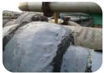
A live leak on a caustic line at a chemical plant required sealing. Previous repairs had failed. The flange fitting was abraded using mechanical grinders and encapsulated using 106 Metal Repair Paste XF
