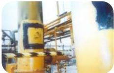
The bottom segment of a chemical process pipe had become badly corroded. The surface of the pipe was mechanically abraded using coarse grinding pads and a pre-formed steel plate cold bonded to the surface.
