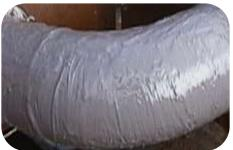
Diesel lines situated on a jetty at a refinery were leaking at the pipe socket. Using handheld scrapers and copper brushes the pipe surface was abraded by hand then coated using 104 Metal Repair Fluid XF
